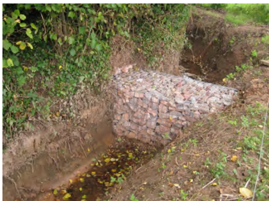
Gabion basket, immediately after construction.
