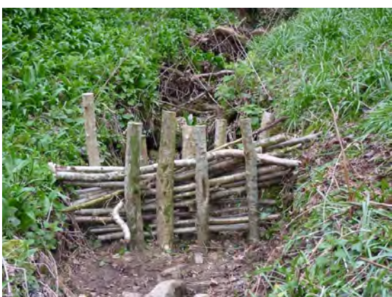
Leaky barrier using hazel bundles
