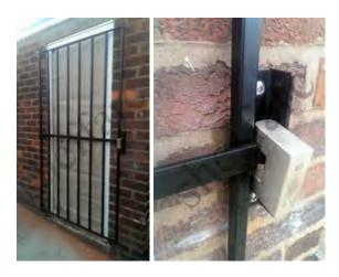
Made from 20mm box section vertical bars, 30mm x 8mm solid bar and 30mmx 30mm angle as a minimum for the horizontals. Fitted with solid steel integral hinges with padlock facility. (single padlock facility as standard).
